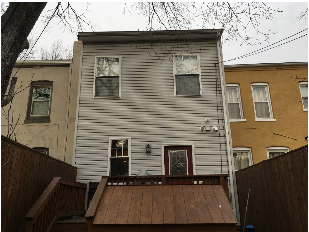
REAR FAÇADE OF 1421 D STREET SE
