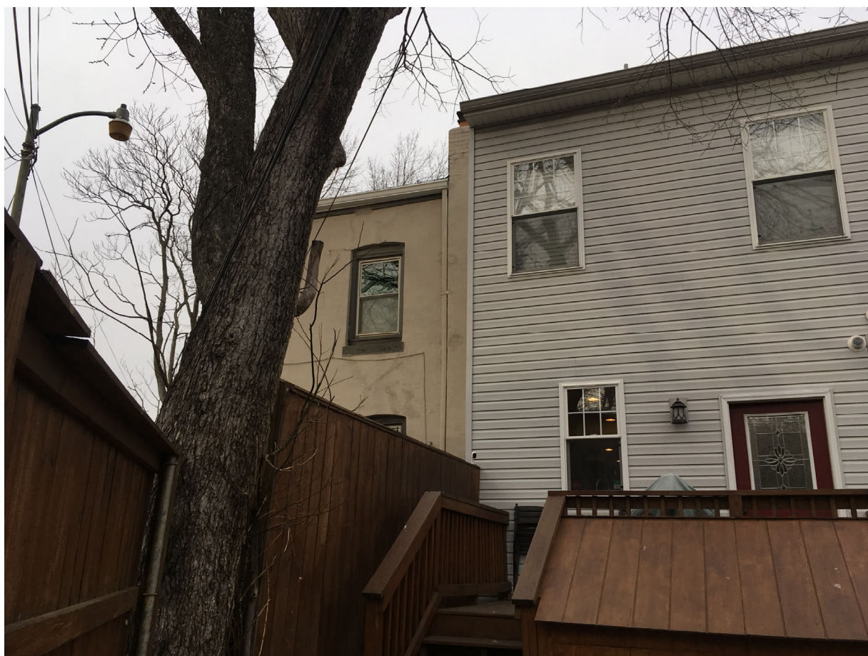
REAR VIEW TOWARDS 1419 D STREET SE
