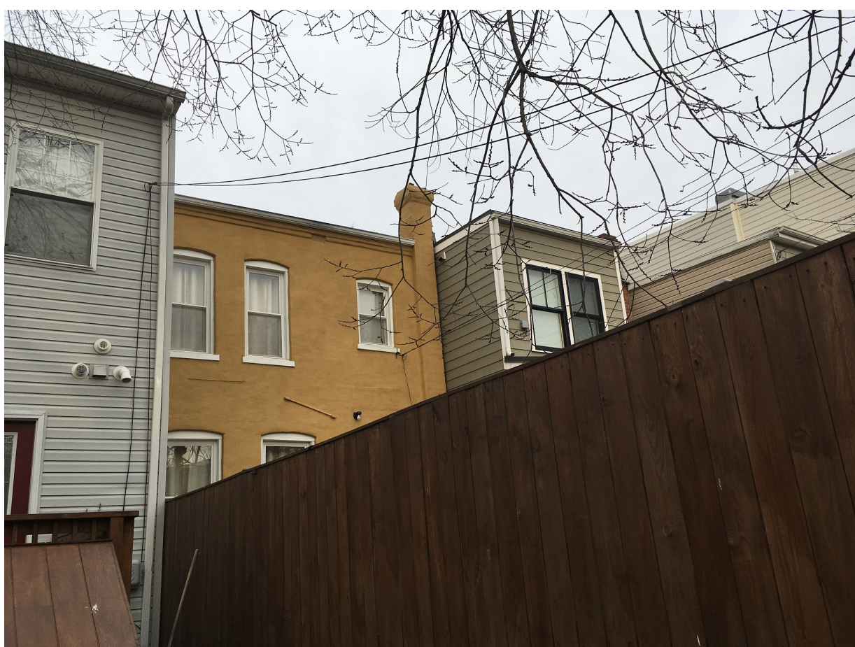
REAR VIEW TOWARDS 1423 D STREET SE
